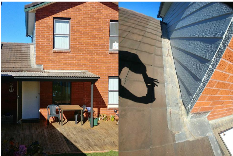
2021 Volcano Art Prize (VAP) Entry. Photographer: Jason Fargie. Title: Beware Lead Flashing on Your Roof Lead-Safety Message: Replace lead flashing with non-lead flashing like Wakaflex, in order to reduce lead in rainwater and stormwater. URL:
